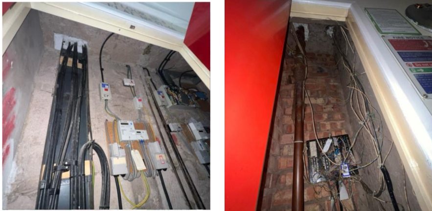
Figure 12 and 13: RC Internal Elements
