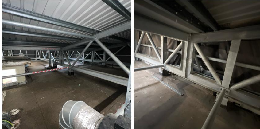
Figure 11 and 12: Lightweight steel frame
