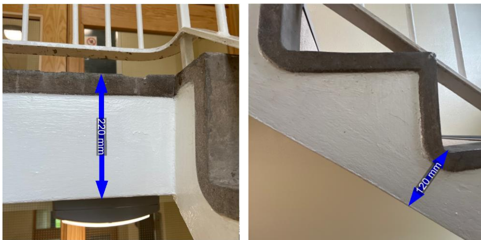
Figure 14 and 15: RC Staircase stringer and slab
