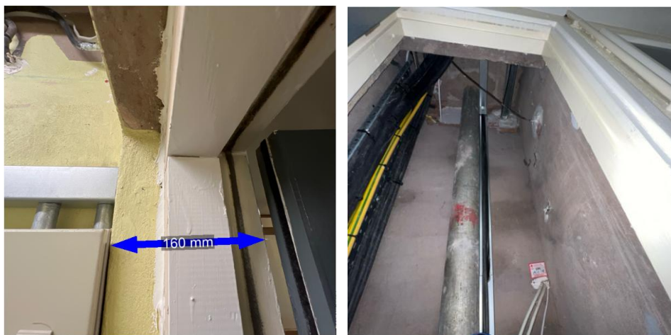
Figure 16 and 17: RC walls
