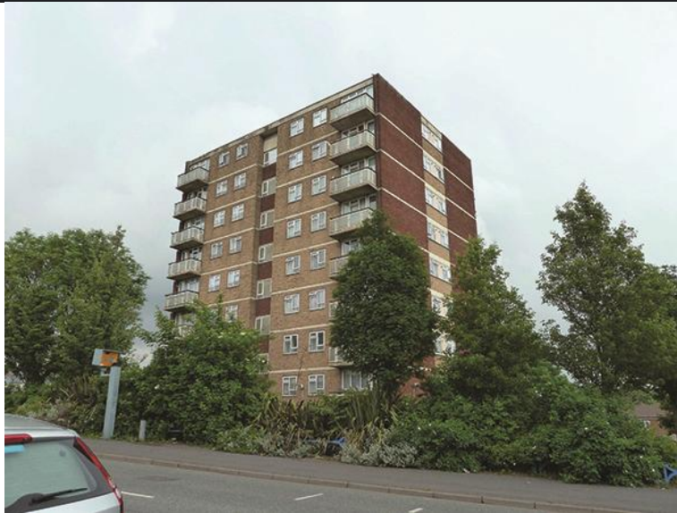
Figure 5. Overview of Nelson House prior to refurbishment
