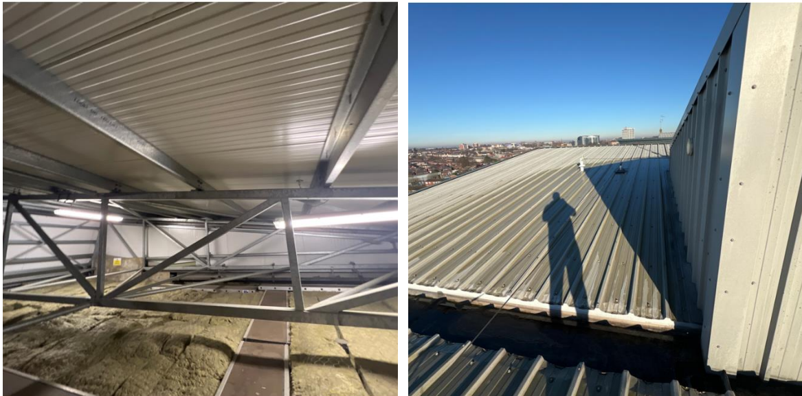
Figure 11 and 12: Roof Level
