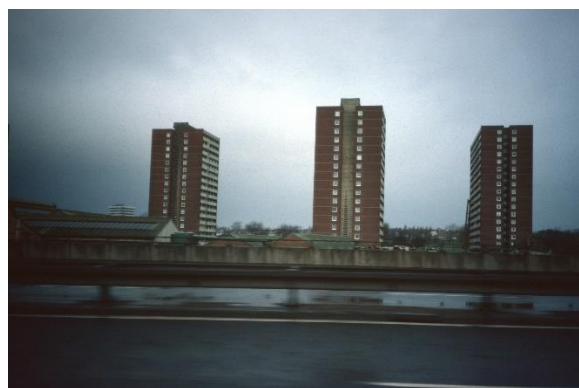
Figure 5. Mountford is the centre building before the refurbishment
