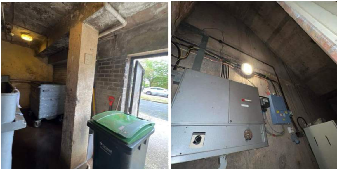
Figure 15 and 16: RC Elements visible within GF Store Rooms
