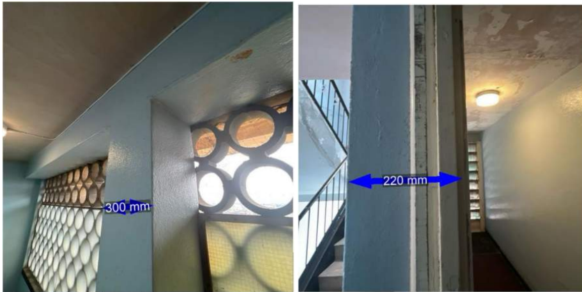
Figure 13 and 14: RC Structure
