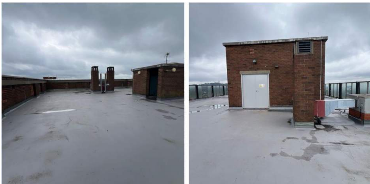
Figure 11 and 12: Roof Level
