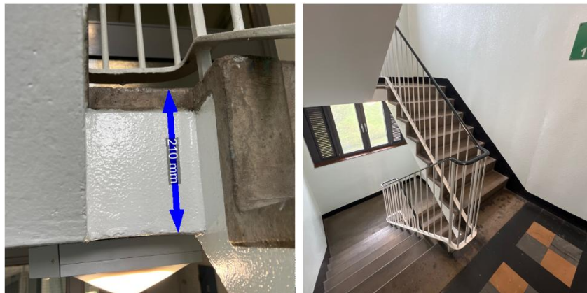
Figure 14 and 15: Stair stringer and Staircase
