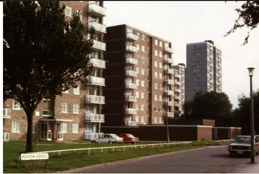
Figure 5. Charlemont Farm estate before the buildings underwent the refurbishment in 2009
