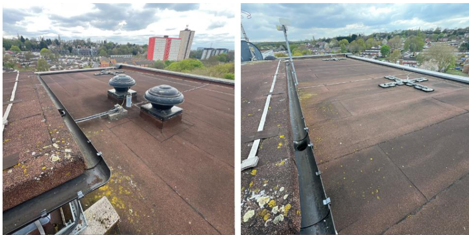
Figure 11 and 12: Roof Level
