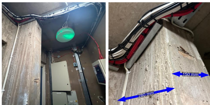
Figure 16 and 17: RC Elements visible
