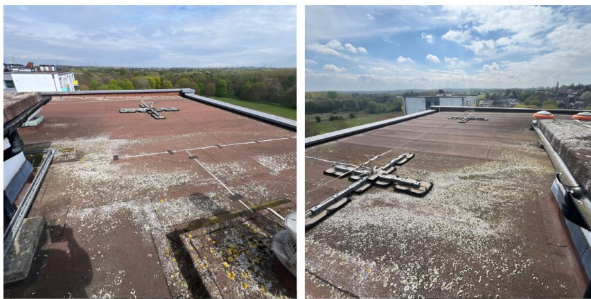
Figure 11 and 12: Roof Level
