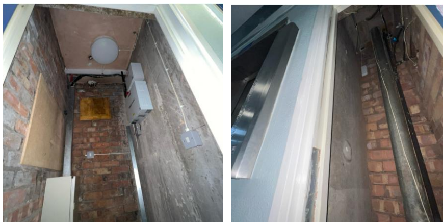
Figure 16 and 17: RC Elements visible
