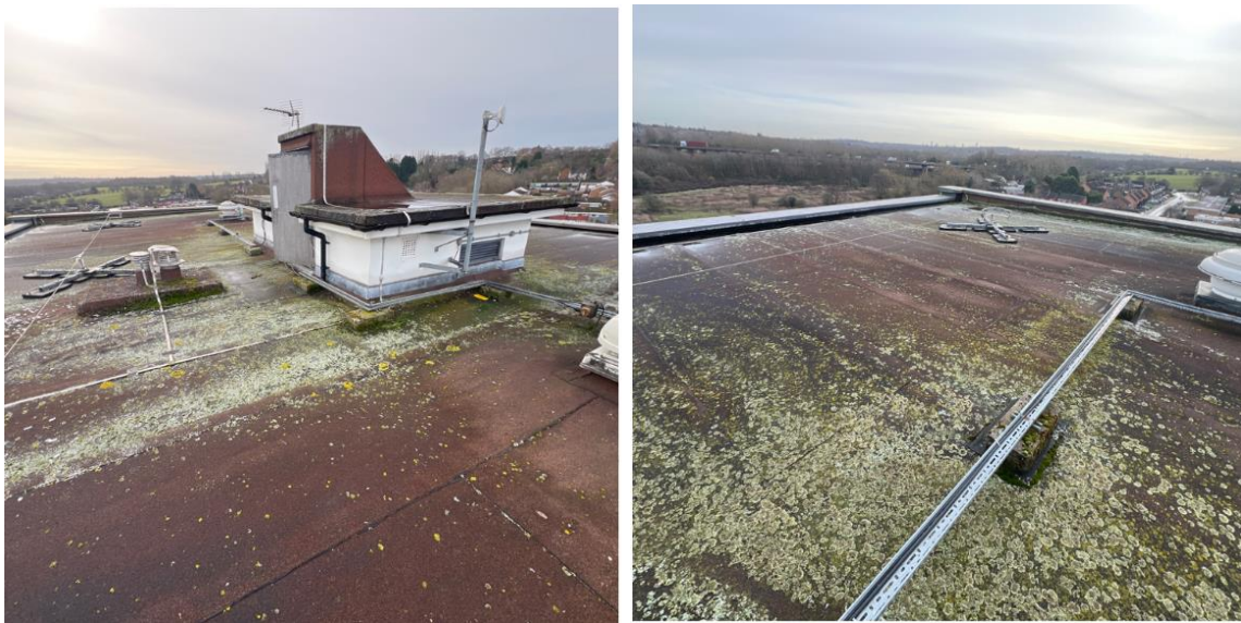
Figure 11 and 12: Roof Level
