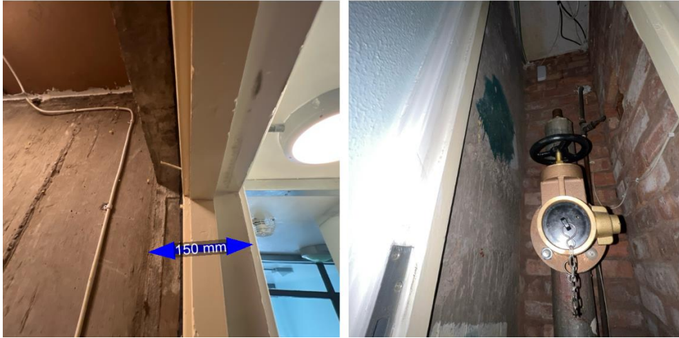
Figure 13 and 14: Vertical RC elements and staircase
