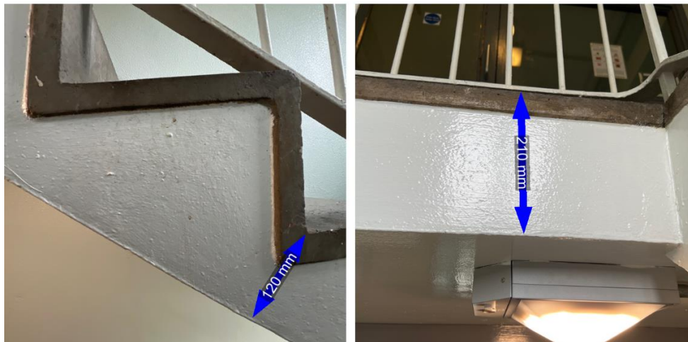
Figure 15 and 16: Stair stringer and RC slab
