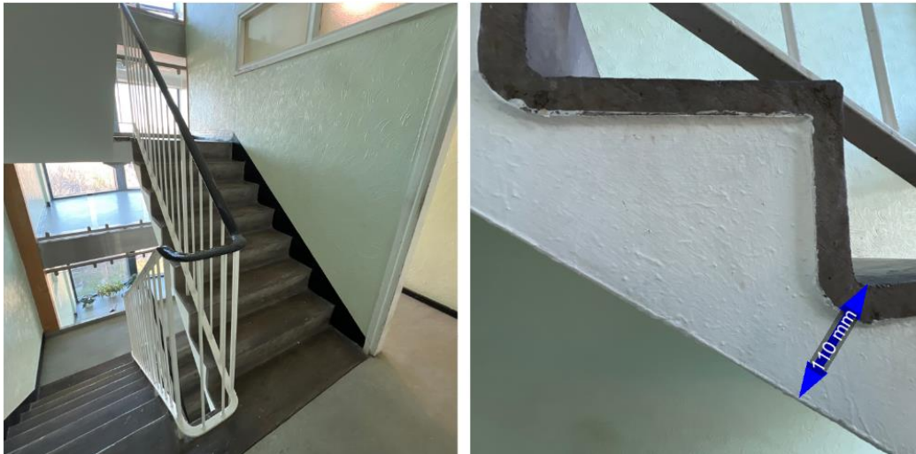
Figure 13 and 14: RC Staircase
