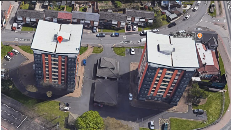
Figure 5. Glover St. before the buildings underwent the refurbishment in 2018
