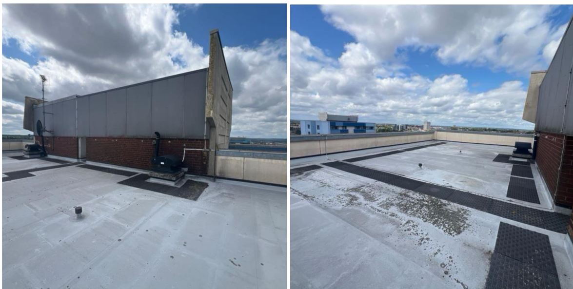
Figure 11 and 12: Roof Level
