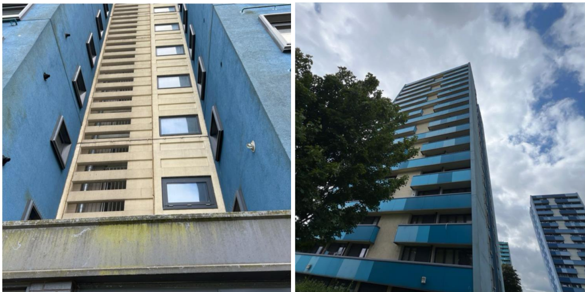
Figure 9 and 10: Precast Panels and side Elevation Balconies
