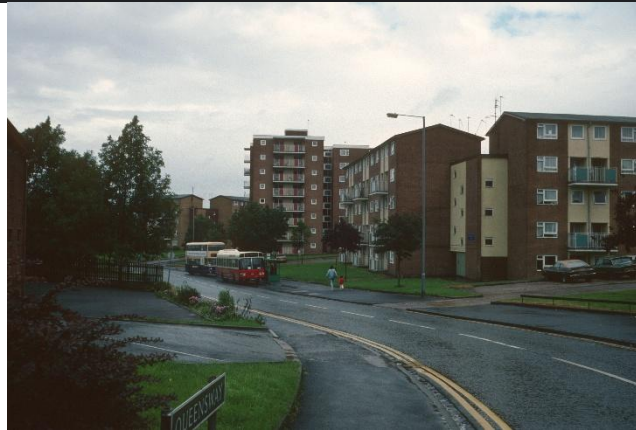
Figure 5. Lawrence Court Prior to Overclad Refurbishment
