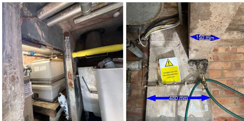
Figure 16 and 17: RC Elements visible at ground floor
