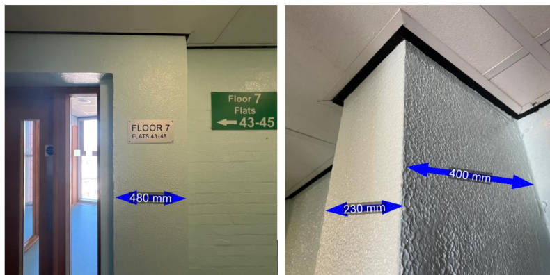
Figure 14 and 15: RC elements at upper floors
