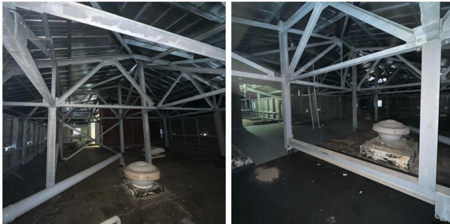
Figure 11 and 12: Roof Level
