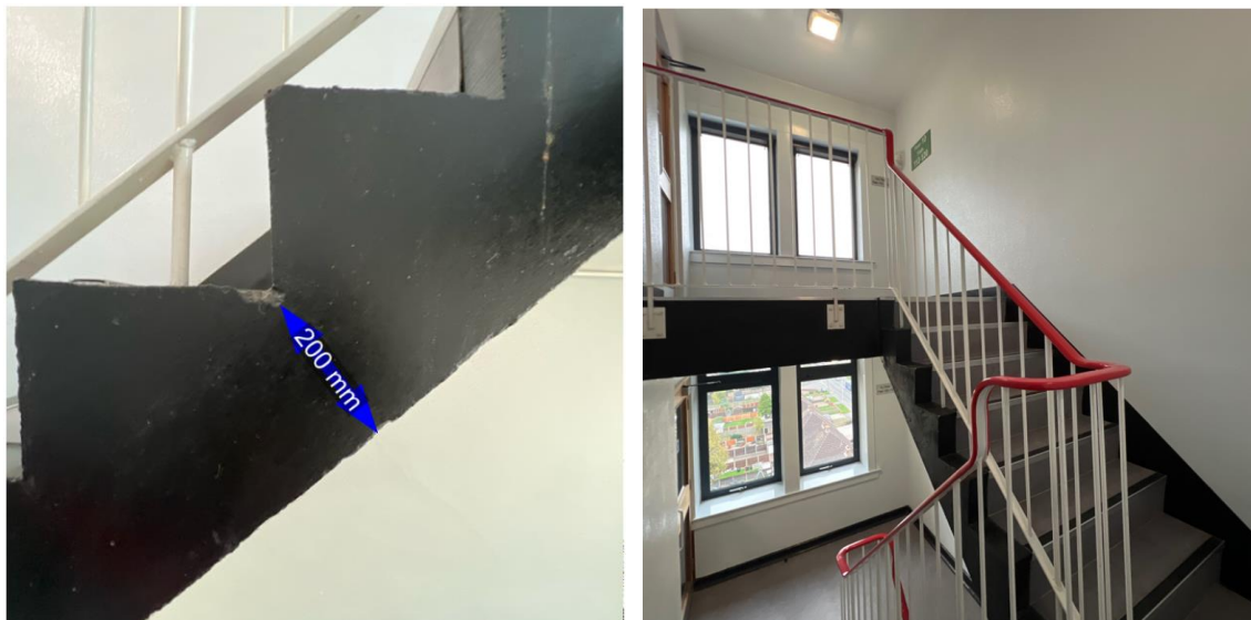
Figure 15 and 16: RC Stringer for staircase
