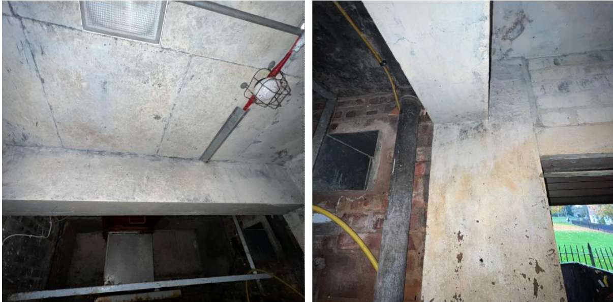
Figure 13 and 14: Structural beams, columns and slab over
