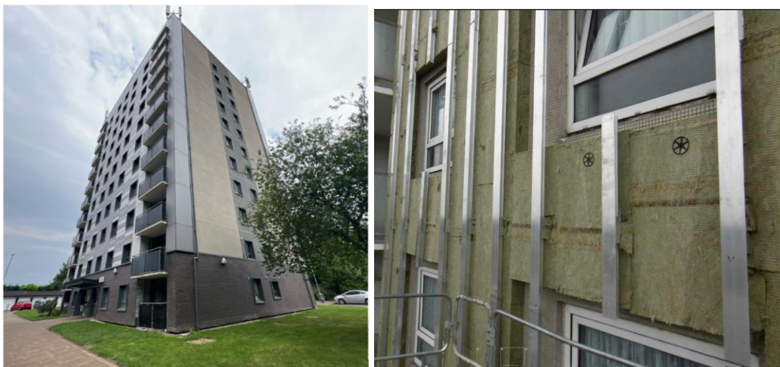
Figure 11 and 12: Building Elevations and photographs of Re-clad in progress
