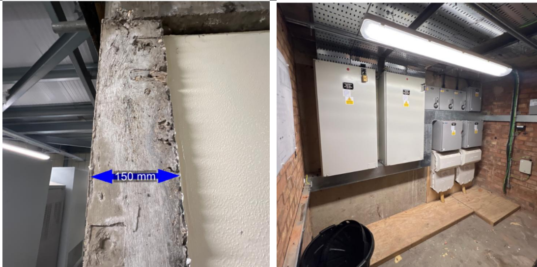
Figure 15 and 16: RC Structure
