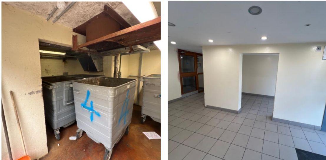
Figure 17 and 18: RC Elements visible and communal areas
