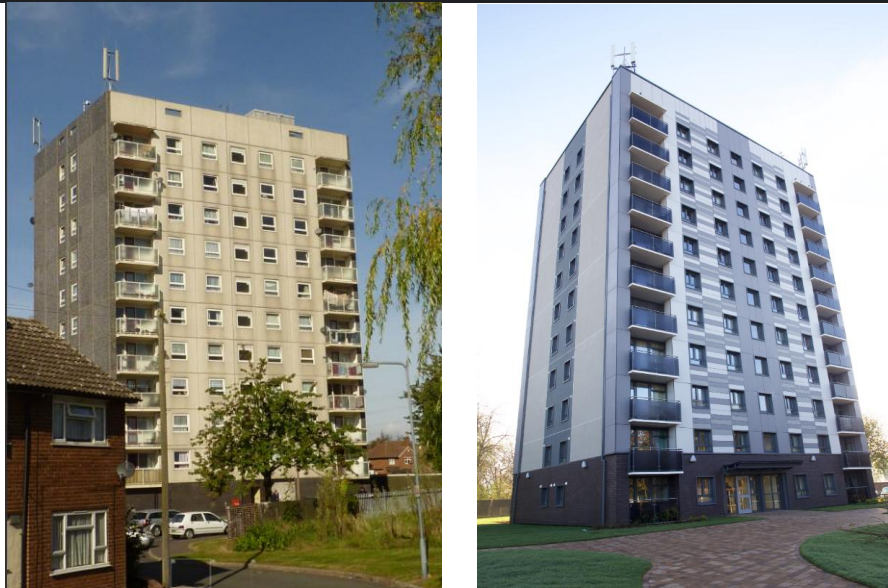
Figure 6 and 7. Archive of the estate photograph from before the overclad
