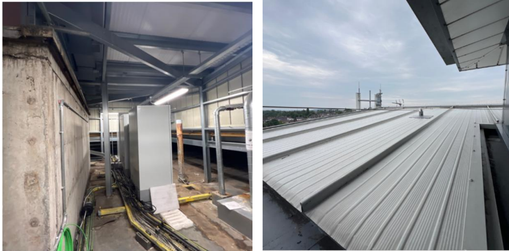
Figure 13 and 14: Roof Level
