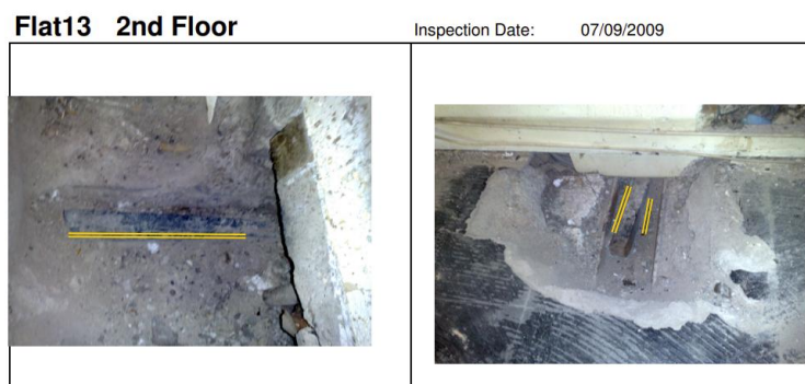
Figure 2: Photographic evidence of ties installed at Russell House. From archive information and historical communications we understand similar stiches between floor slabs and external walls are installed at Kynaston also, however we have no evidence. Therefore some intrusive investigations required to evidence their presence.
