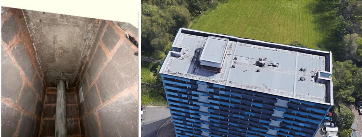
Figure 11 and 12: Underside of roof slab and satellite image
