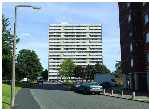
Figure 5. Building Before Refurbishment
