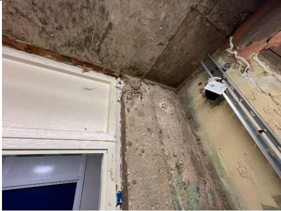
Figure 13 and 14: Localised spalling and Vertical RC Structure Visible in Bin Store
