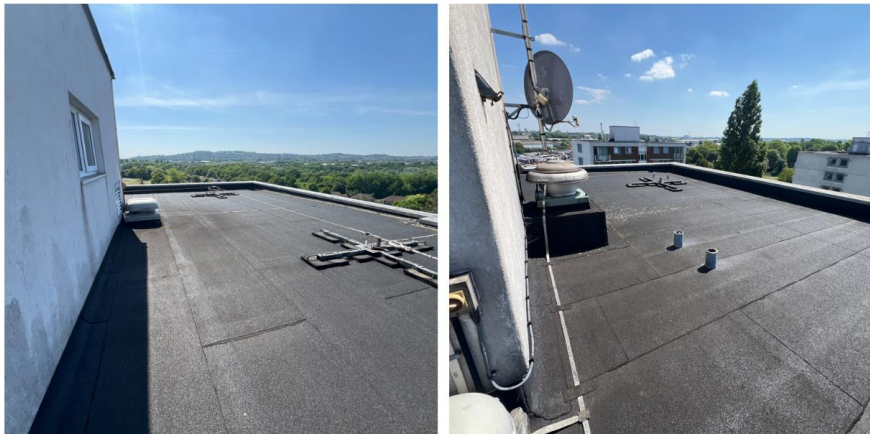
Figure 11 and 12: Roof Level
