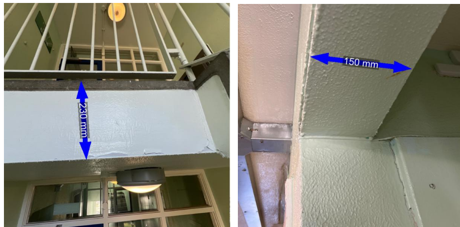
Figure 16 and 17: Slab Edge and wall thickness
