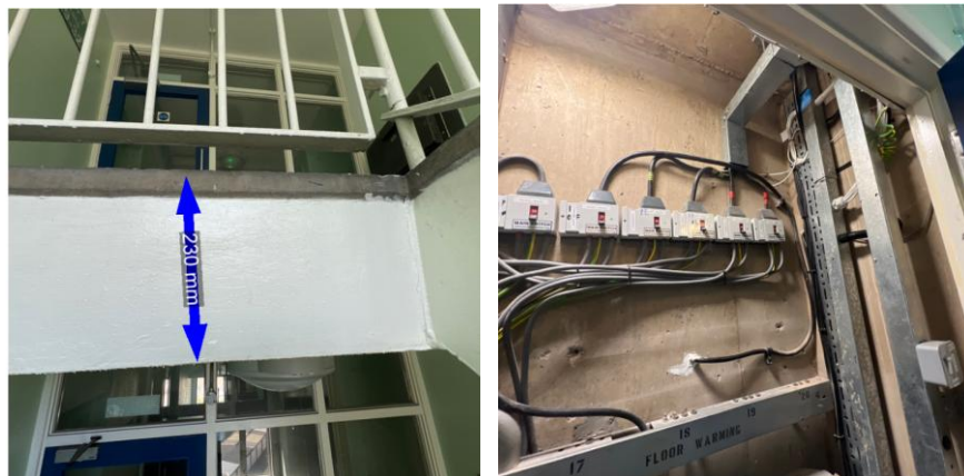
Figure 16 and 17: Slab Edge and stability wall
