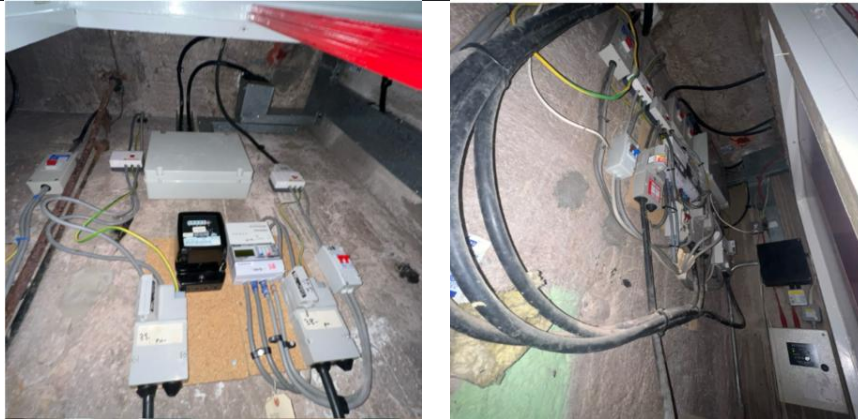
Figure 12 and 13: RC Internal Elements
