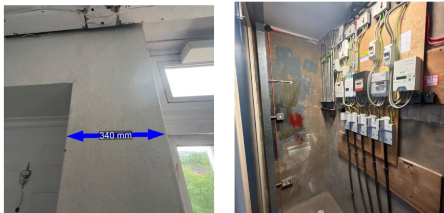
Figure 16 and 17: RC internal elements
