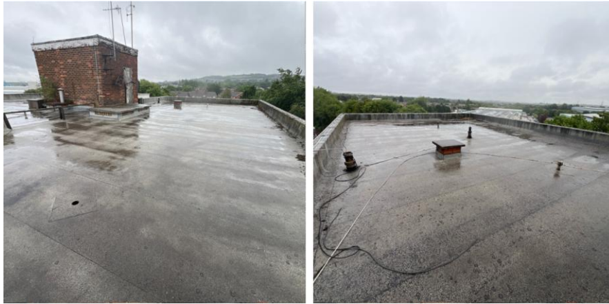
Figure 11 and 12: Roof Level
