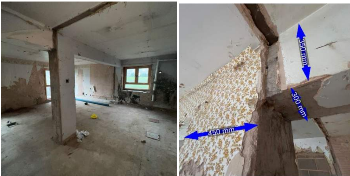
Figure 15 and 16: RC Elements visible with GF Store Rooms
