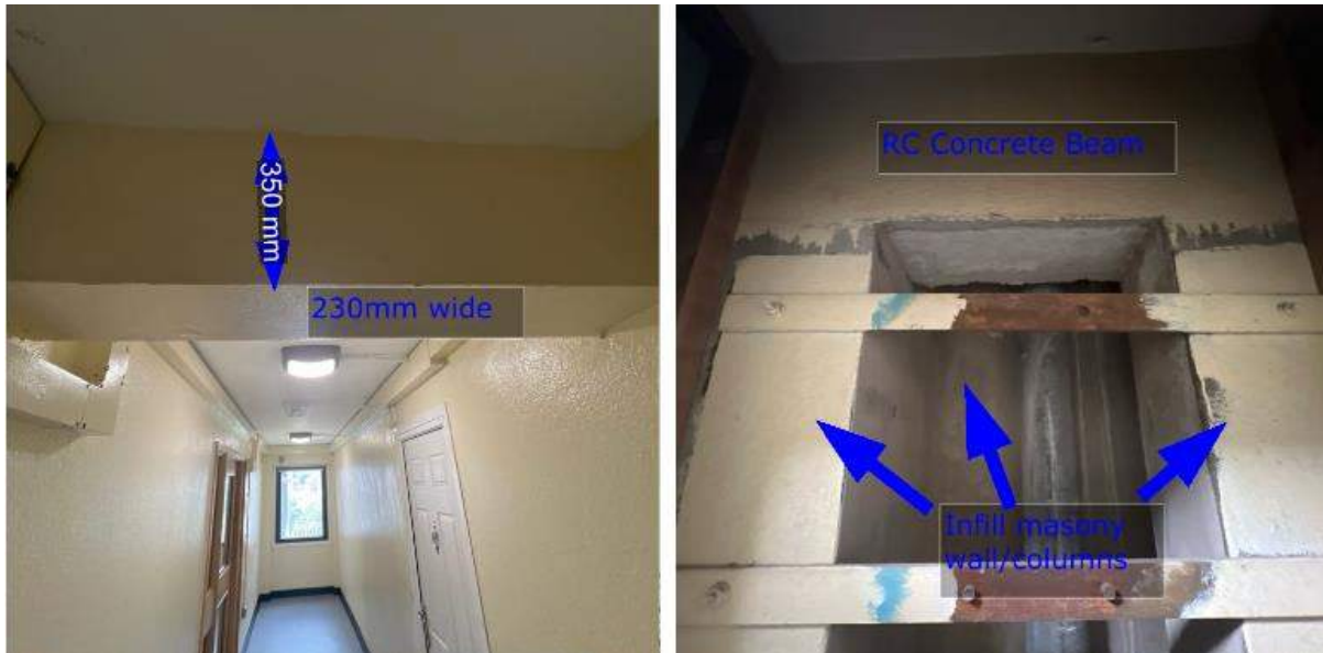
Figure 13 and 14: RC Structure
