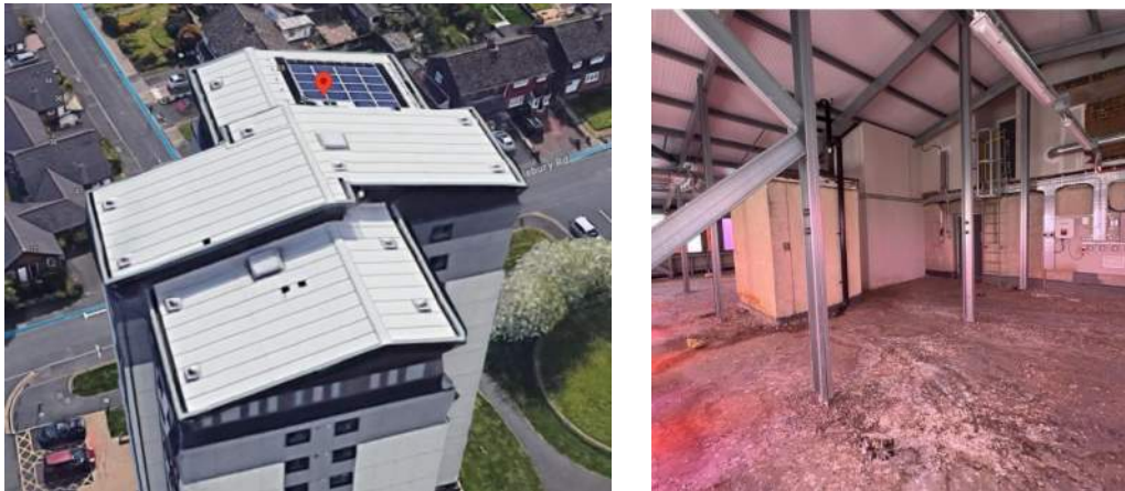
Figure 11 and 12: Roof Level
