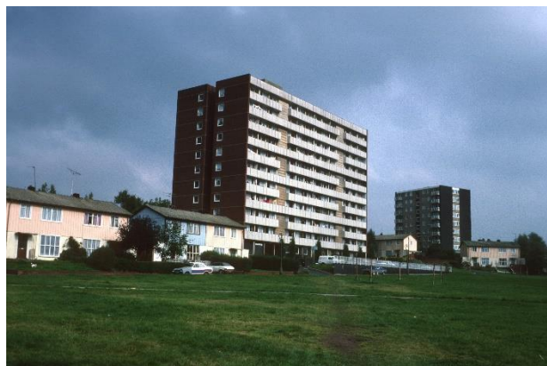
Figure 5. Building in before refurbishment
