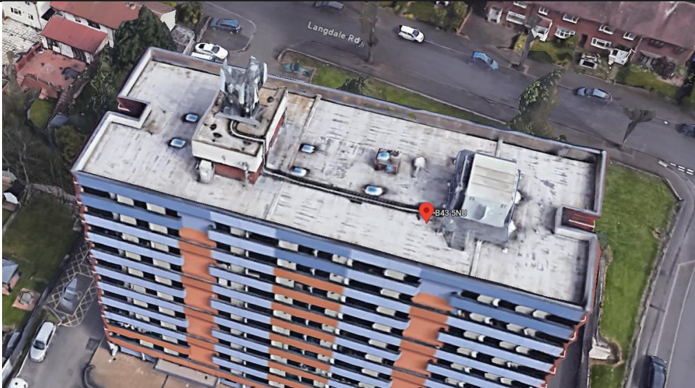
Figure 11: Roof level enclosure
