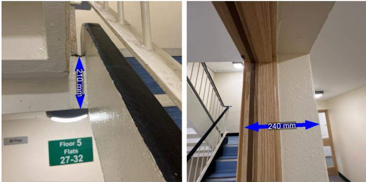
Figure 13 and 14: Stair stringer and concrete frame
