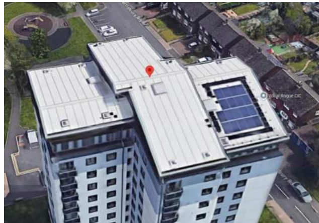
Figure 11 and 12: Roof Level
