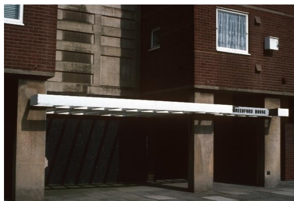
Figure 5. Greenford is building to the front before refurbishment
