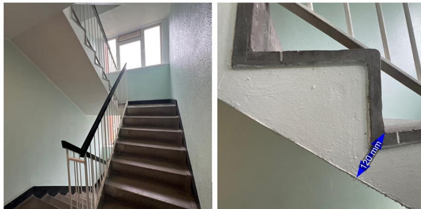
Figure 14 and 15: Stair stringer and Staircase
