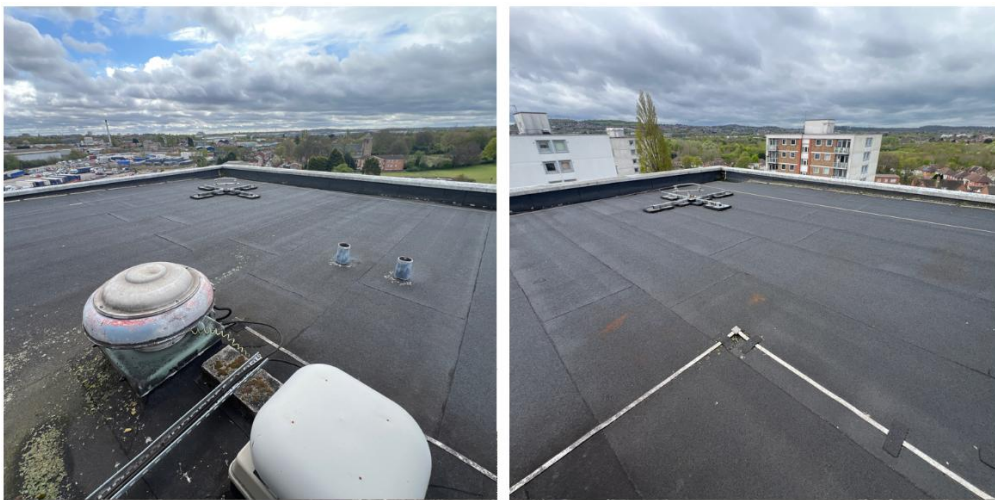
Figure 11 and 12: Roof Level
