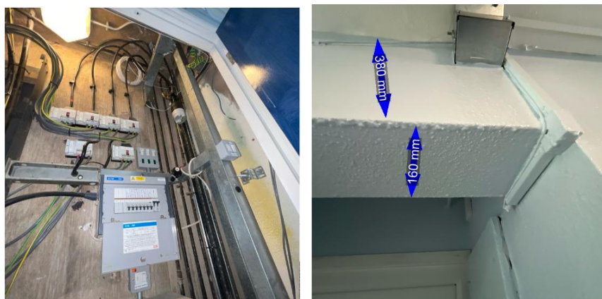
Figure 16 and 17: RC Elements visible
