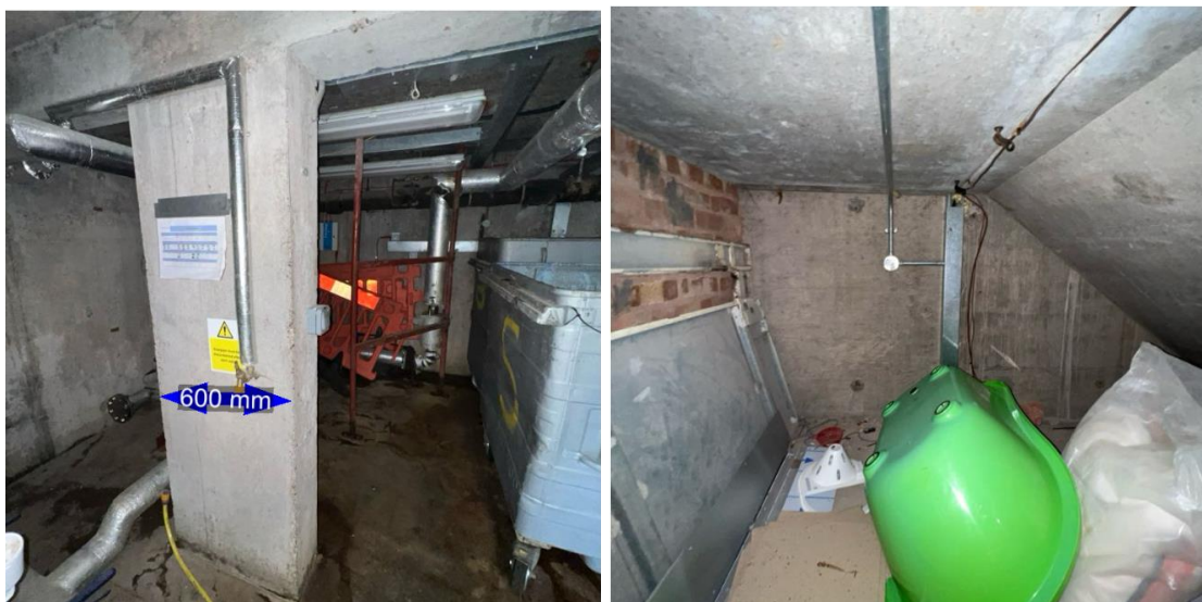
Figure 15 and 16: RC Elements visible within basement level which covers partial footprint.
