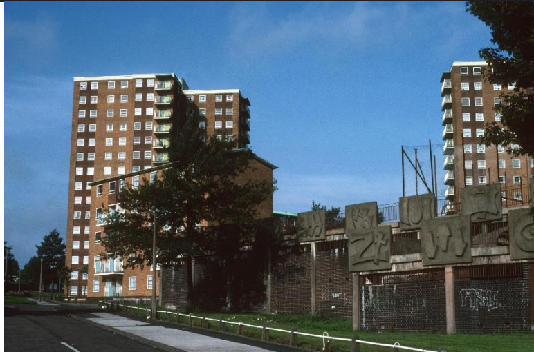
Figure 5. Estate before the buildings underwent the refurbishment in 2016
