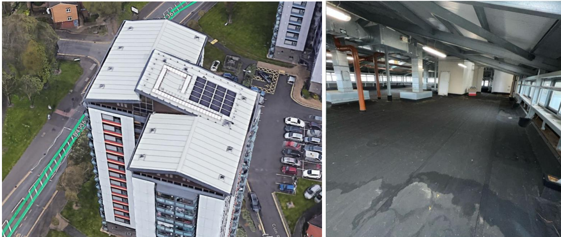
Figure 11 and 12: Roof Level
