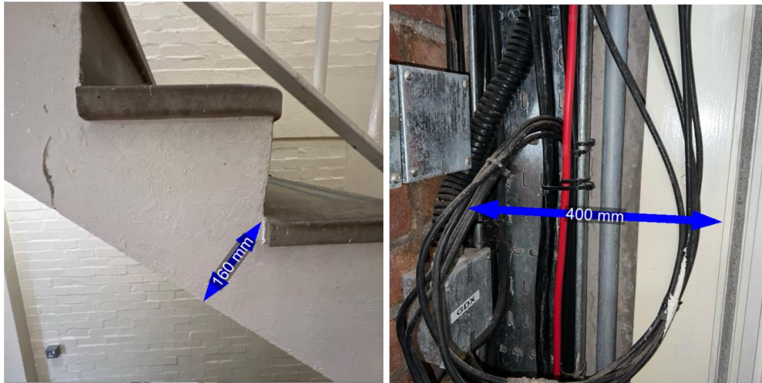
Figure 13 and 14: Stair stringer and size of concrete columns
