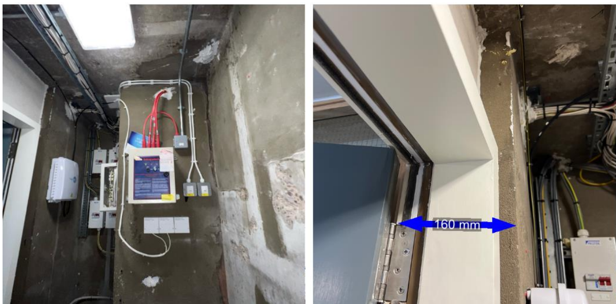
Figure 15 and 16: RC Elements visible at ground floor
