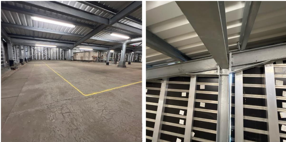
Figure 11 and 12: Roof Level
