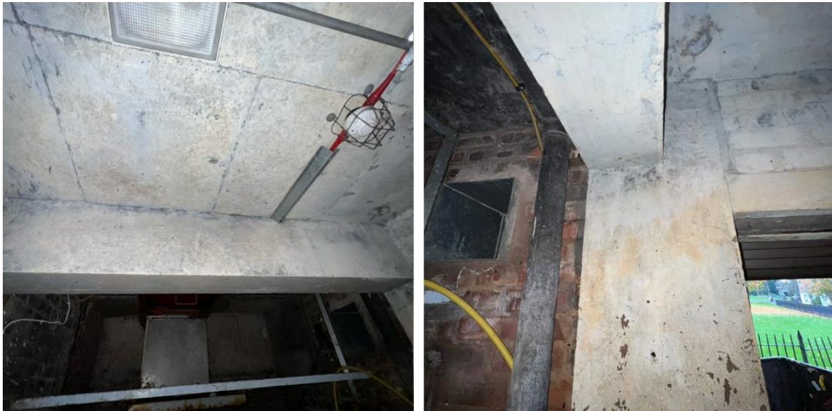
Figure 13 and 14: Structural beams, columns and slab over
