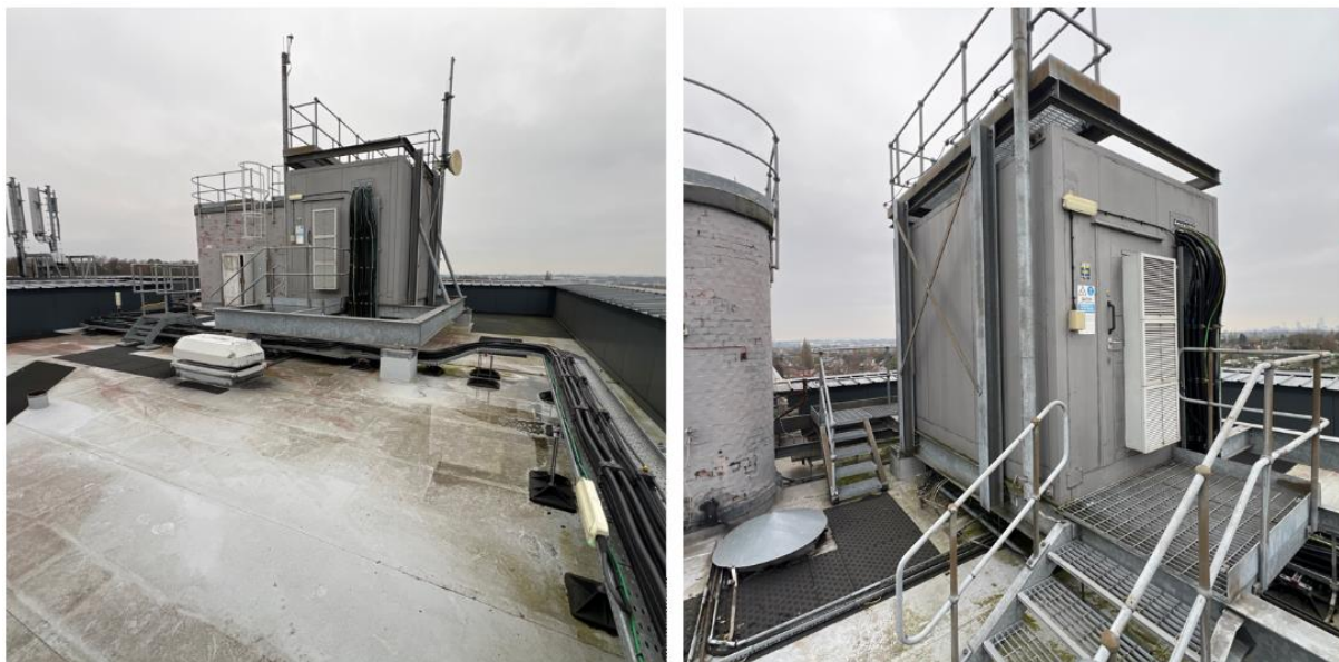
Figure 11 and 12: Roof Level
