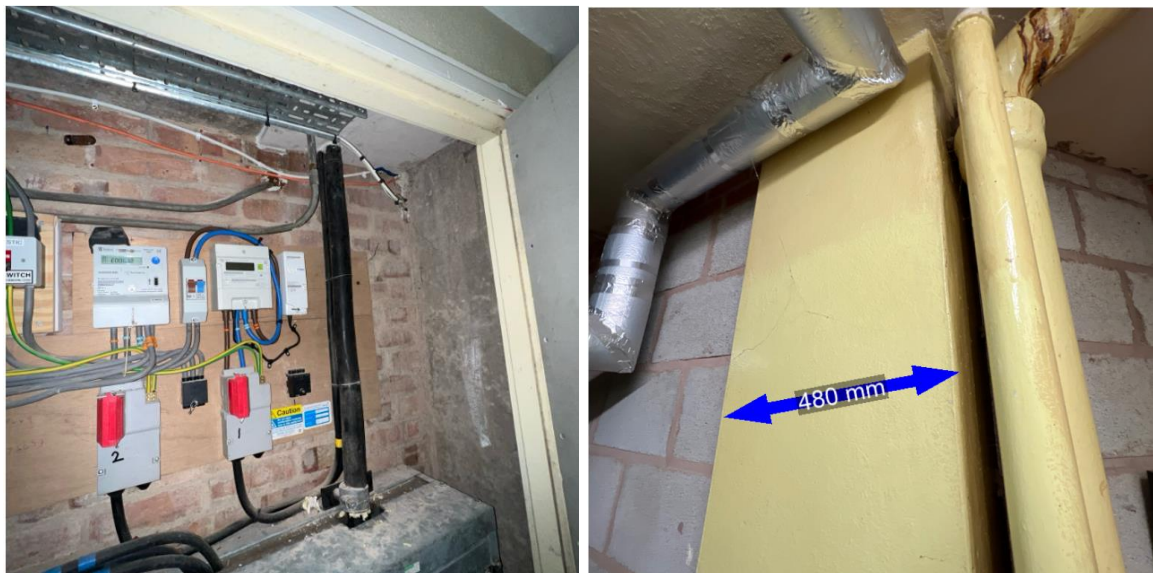
Figure 15 and 16: RC Elements visible within Service cupboards and water tank room
