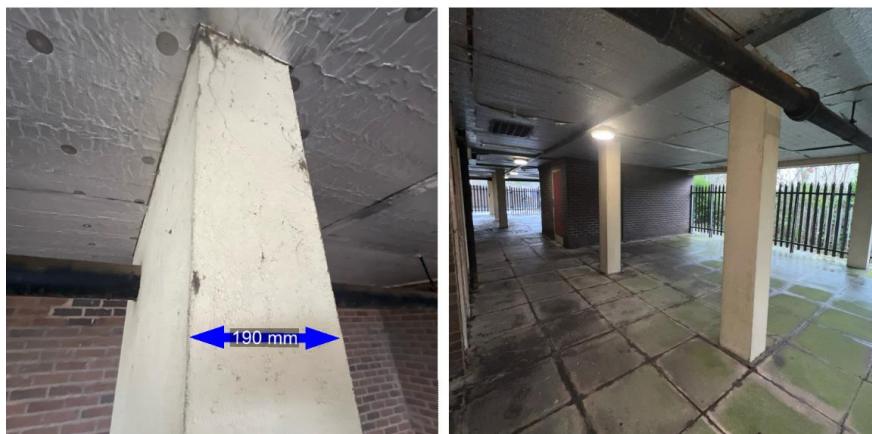
Figure 12 and 13: Vertical RC Structure Visible
