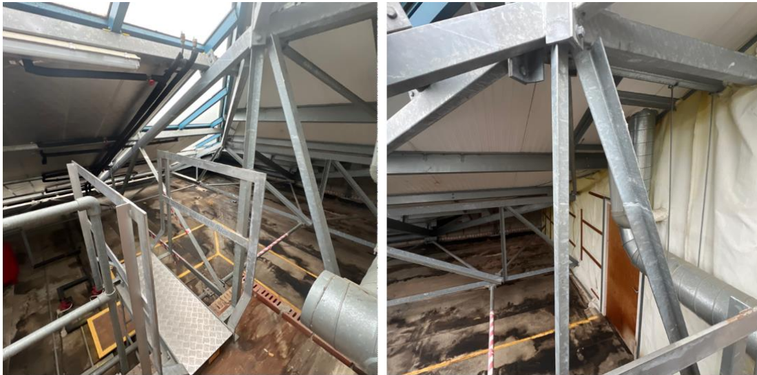
Figure 11 and 12: Roof Level
