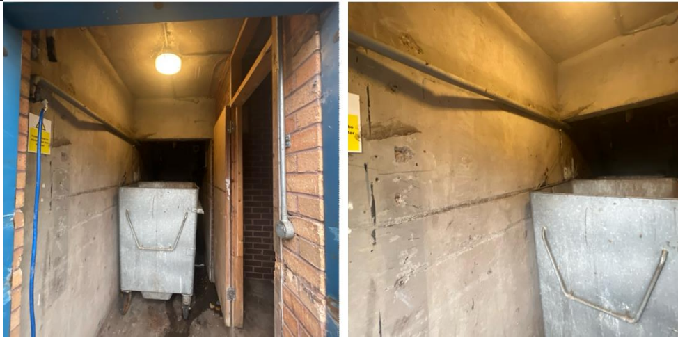
Figure 13 and 14: Structural beams, columns and slab over
