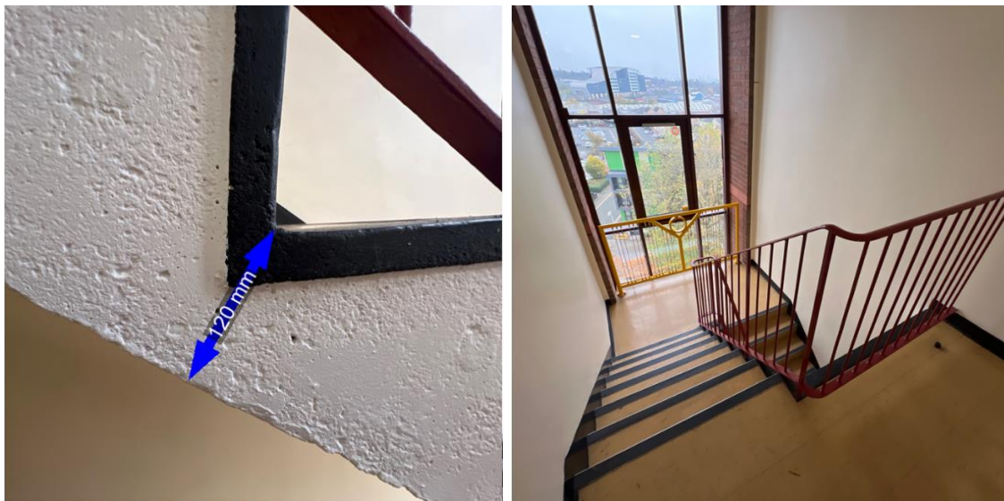
Figure 15 and 16: RC Stringer for staircase
