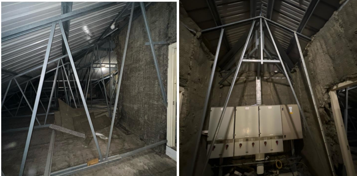
Figure 11 and 12: Roof Level
