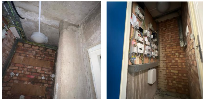
Figure 16 and 17: RC internal elements
