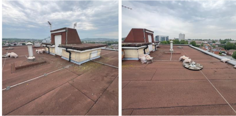
Figure 11 and 12: Roof Level
