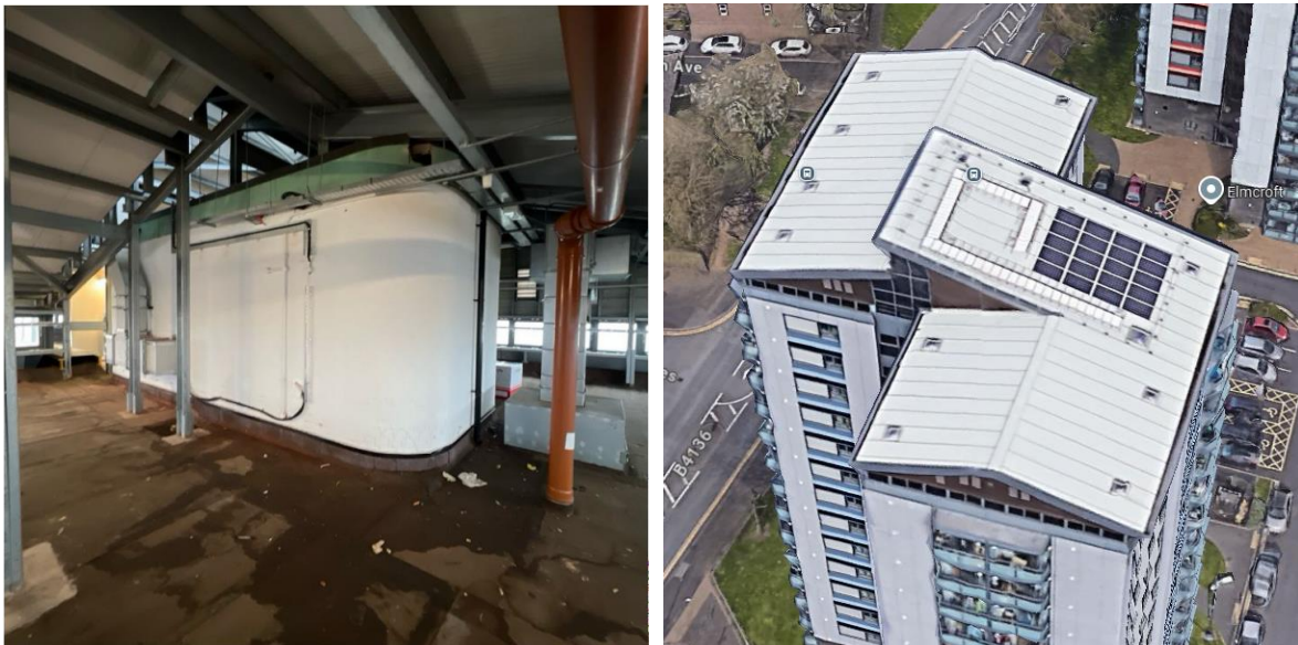
Figure 11 and 12: Roof Level
