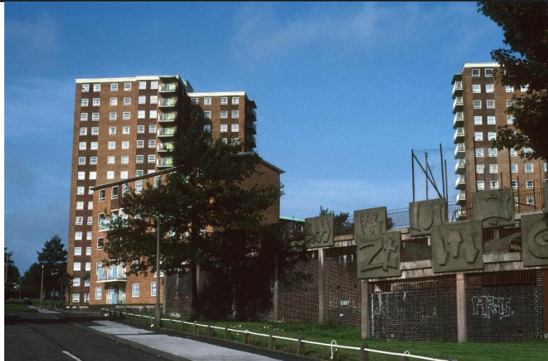
Figure 5. Neighbouring Property before the buildings underwent the refurbishment in 2016
