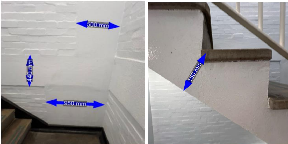
Figure 13 and 14: Stair stringer and concrete frame
