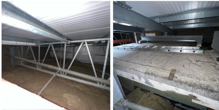
Figure 11 and 12: Roof Level
