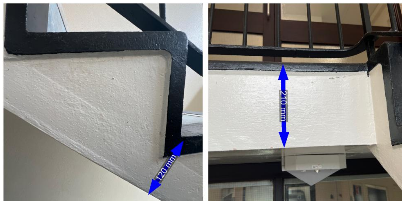
Figure 14 and 15: Stair stringer and concrete slab
