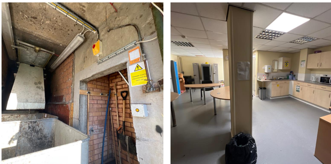
Figure 15 and 16: RC Elements visible at ground floor
