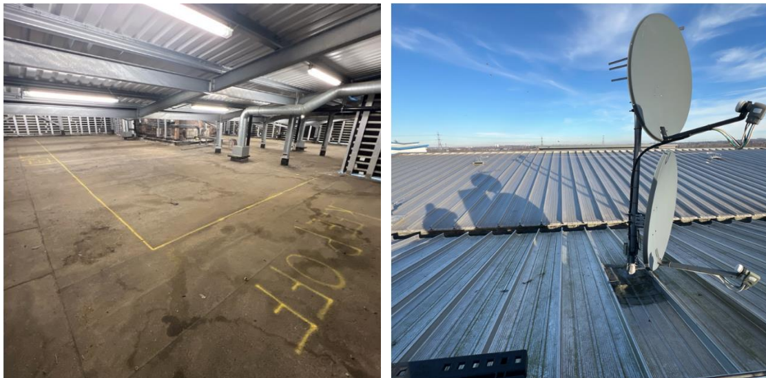
Figure 11 and 12: Roof Level
