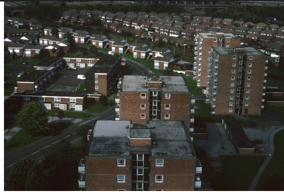
Figure 5. Charlemont Farm estate before the buildings underwent the refurbishment in 2015
