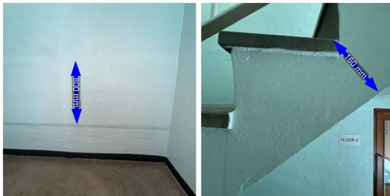
Figure 14 and 15: Stair stringer and concrete element
