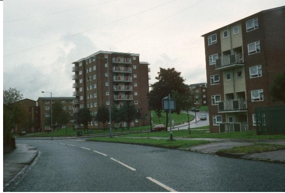
Figure 5. Astbury Court Prior to Overclad Refurbishment
