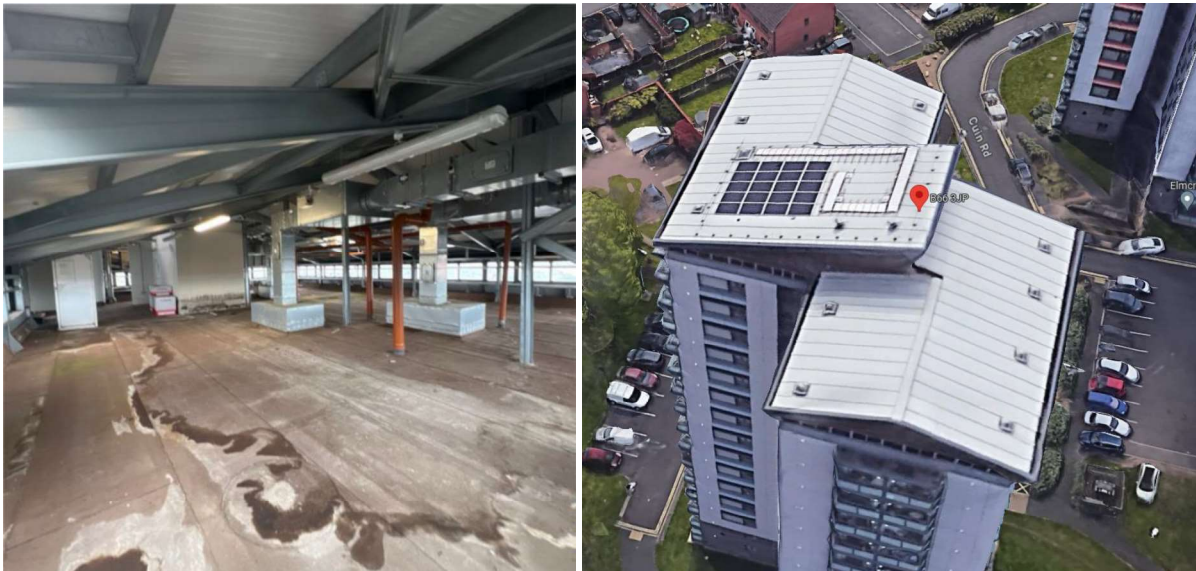
Figure 11 and 12: Roof Level
