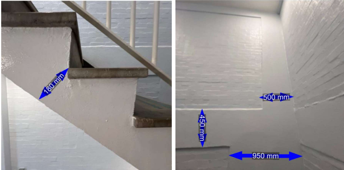
Figure 13 and 14: Stair stringer and concrete frame
