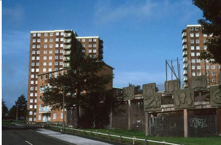
Figure 5. Neighbouring Property before the building underwent the refurbishment in 2016
