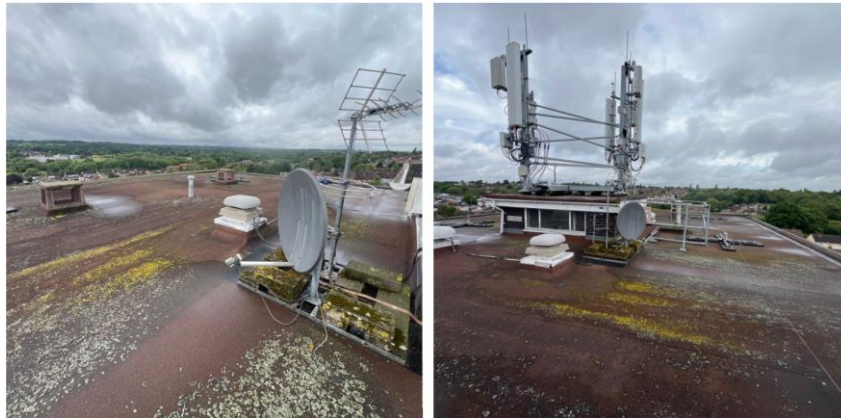
Figure 11 and 12: Roof Level
