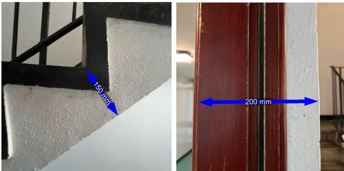
Figure 14 and 15: Staircase Stringer and shear wall
