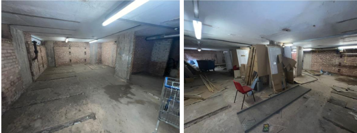
Figure 12 and 13: Vertical RC Structure Visible
