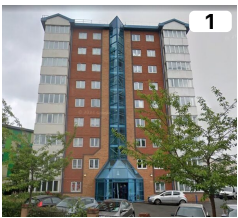
West Elevation (Front Entrance)
