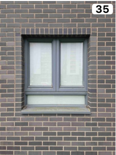
Top, Mid, Side Hung Casements (FSRVBN)
