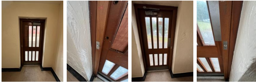
Final exit doors and access release.
