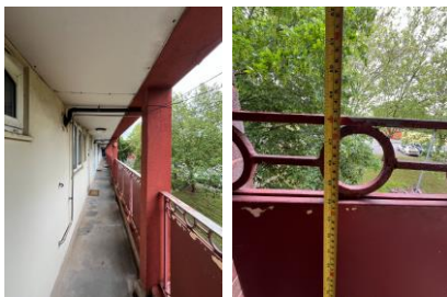
1 st floor open deck railings
