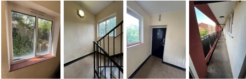
1st and 2 nd floor landing
