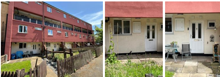
Ground floor flats 1-6
