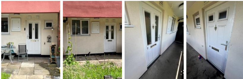
Ground & 1 st Floor flats entrance doors
