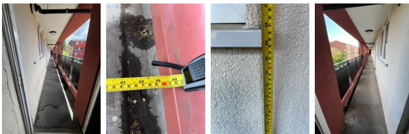
1 st floor open deck with width and height of windows
