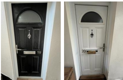
Ground floor flats 19,20
