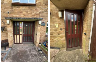
Front and rear entrances to block
