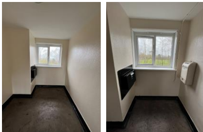
1 st and 2 nd floor landing
