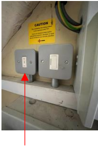
Emergency light test switch
