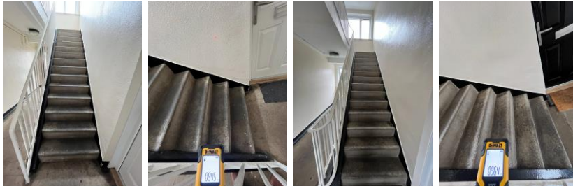
Ground to 1 st & 2 nd floor staircase.
