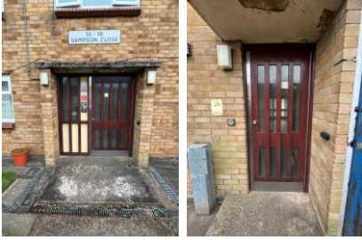
Front and rear entrances to block
