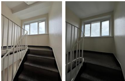
1 st and 2 nd floor landing
