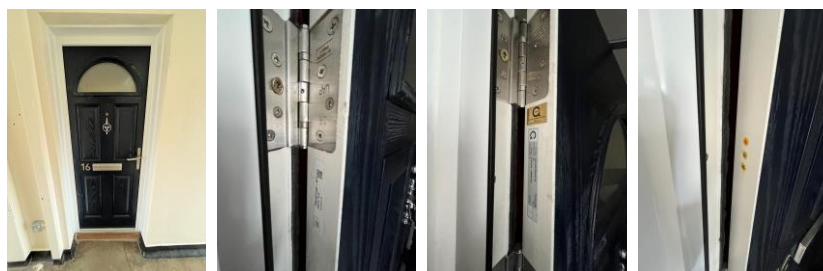
Confirmation of Certified Composite FD30s at flat 16
