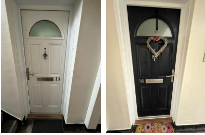
Ground floor flats 13,14
