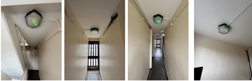
Communal corridors on ground, 1 st and 2 nd floors
