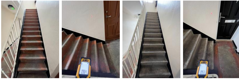
Ground to 1 st & 2 nd floor staircase.
