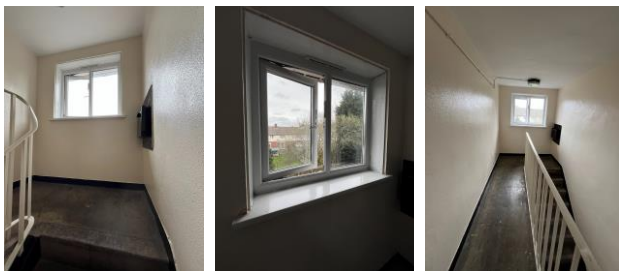
1st and 2 nd floor landing
