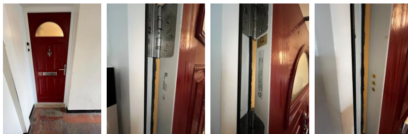
Confirmation of Certified Composite FD30s at flat 10
