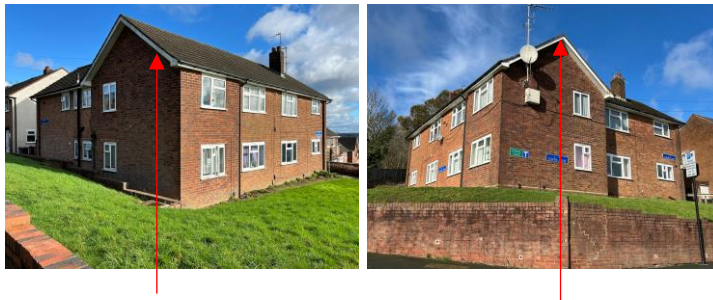
Laminated boards on the underside & fascia
