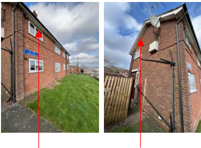
Laminated boards on the underside & fascia
