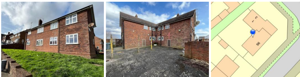
96-96A Tower Road front and rear
