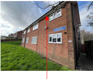
Laminated boards on the underside & fascia
