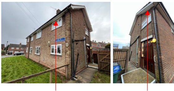
Laminated boards on the underside & fascia
