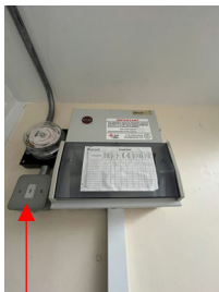
Emergency lights test switch
